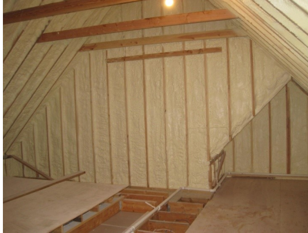
Figure 34: Grade I Closed-Cell Spray Foam – Exterior Walls
