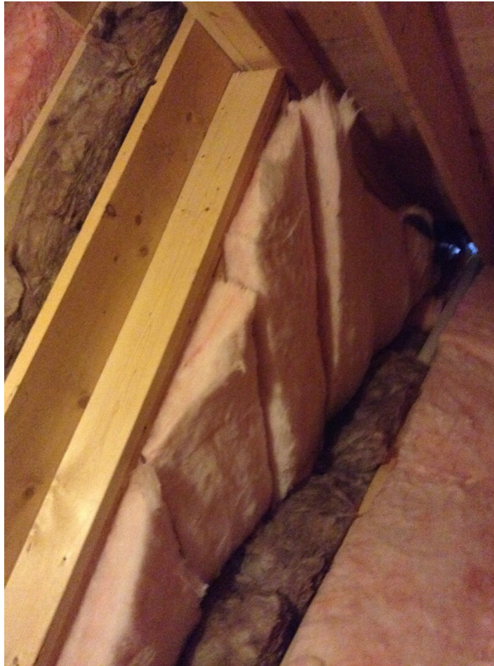
Figure 36: Grade III Fiberglass Batts – Attic Kneewalls
