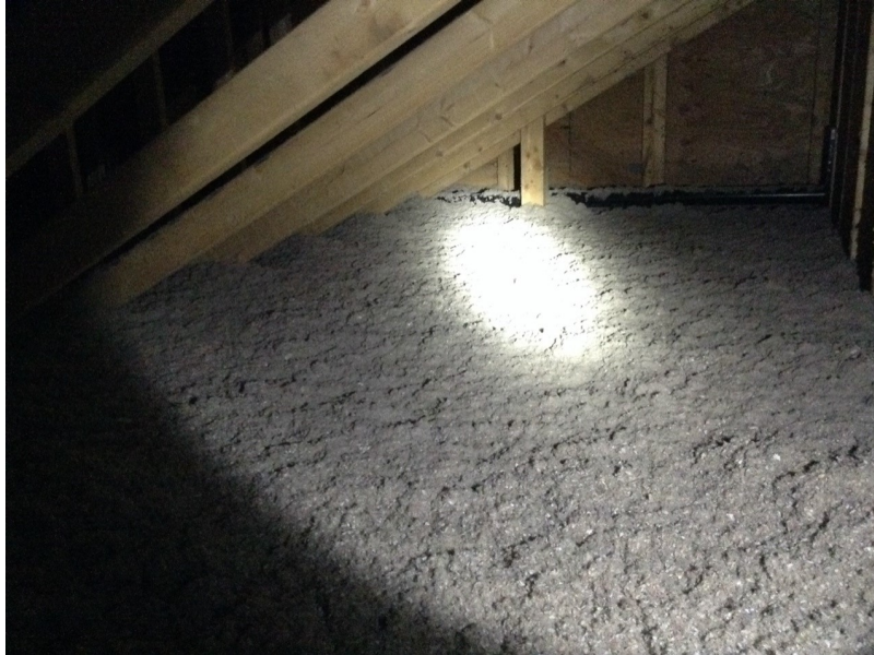
Figure 39: Grade I Blown Cellulose – Attic
