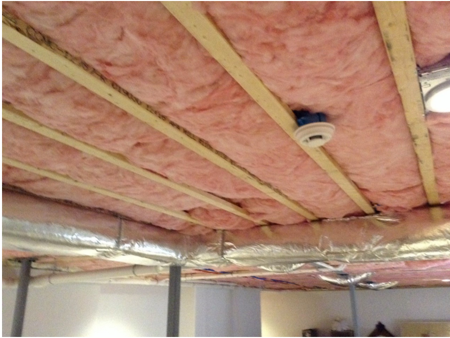
Figure 37: Grade II Fiberglass Batts – Frame Floor
