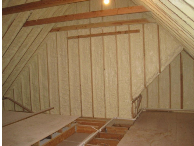
Figure 35: Grade I Closed-Cell Spray Foam – Exterior Walls
