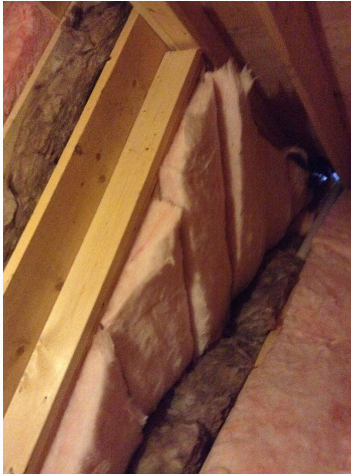
Figure 37: Grade III Fiberglass Batts – Attic Knee Walls
