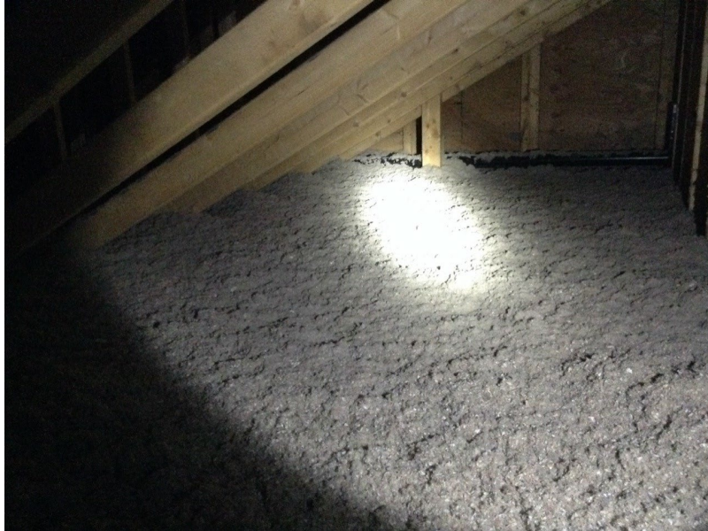
Figure 40: Grade I Blown Cellulose – Attic
