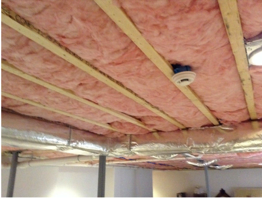
Figure 38: Grade II Fiberglass Batts – Frame Floor
