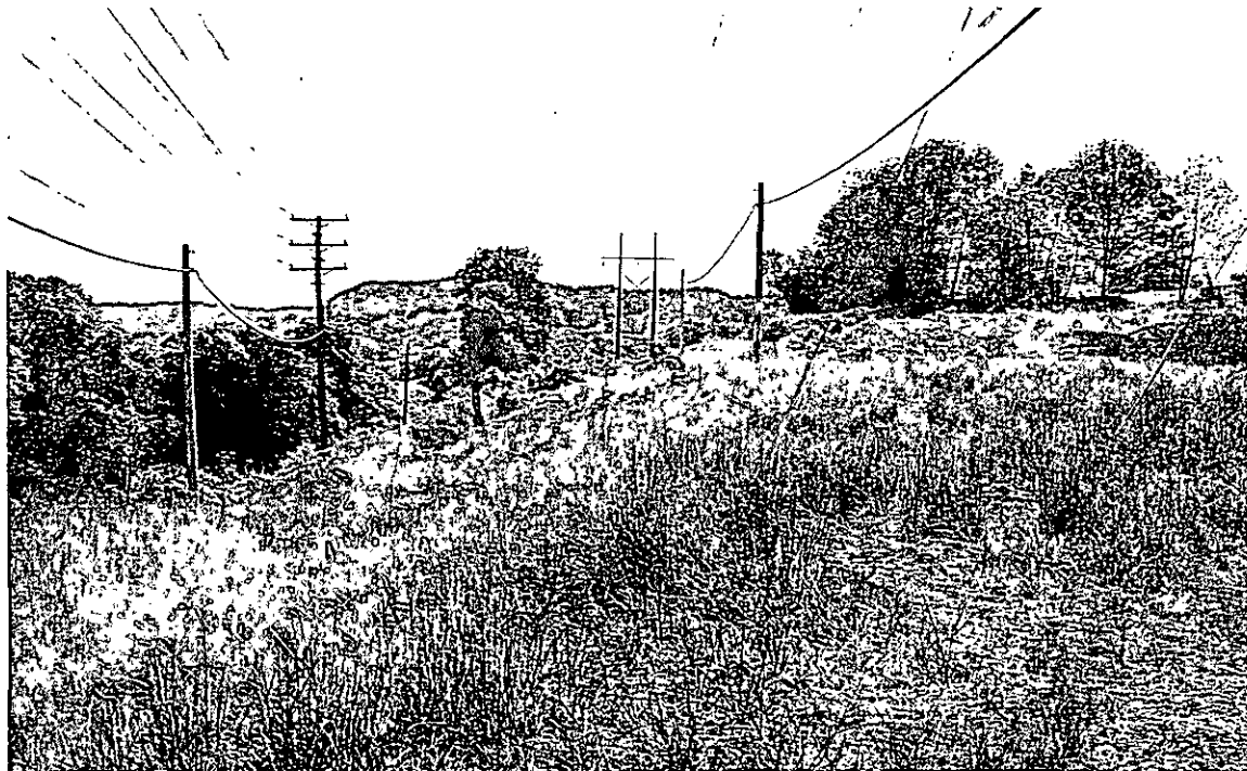
Photograph 7. Existing Line #1 Proceeding Eastward on a Wooded Ridge above the Allegheny River
