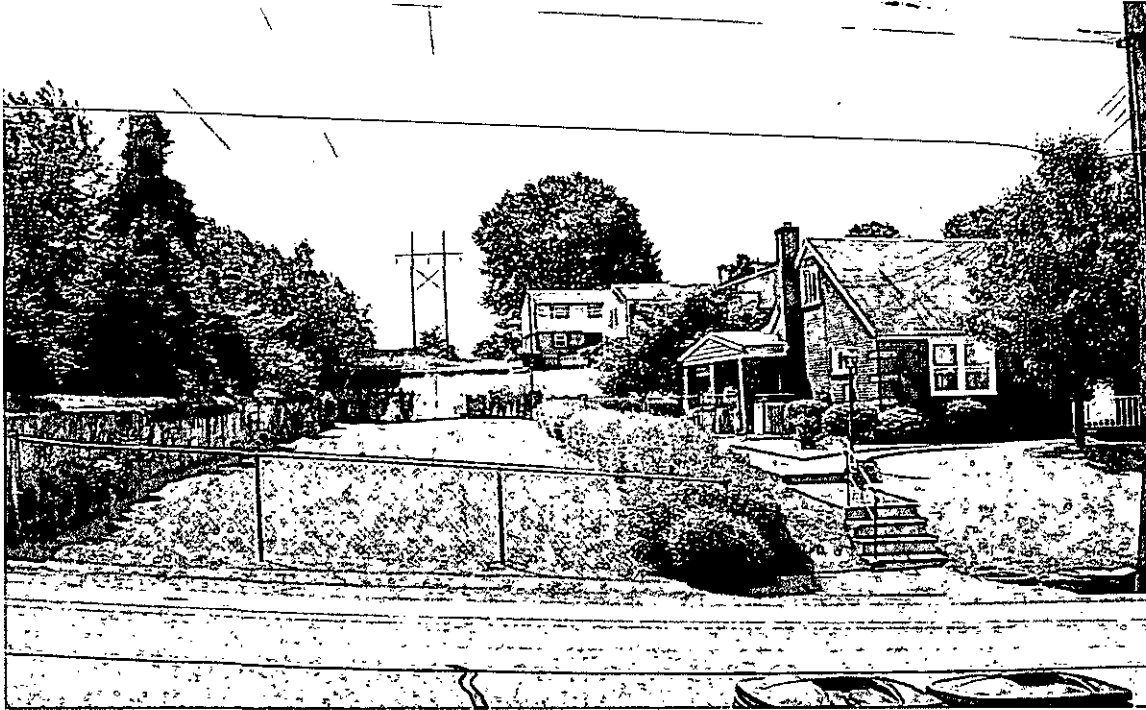
Photograph 5. Existing Line #1 as it Proceeds Along Side Yards of Penn Hills Neighborhood
