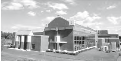
State-of-the-art Pickering Water Treatment Plant comes online
