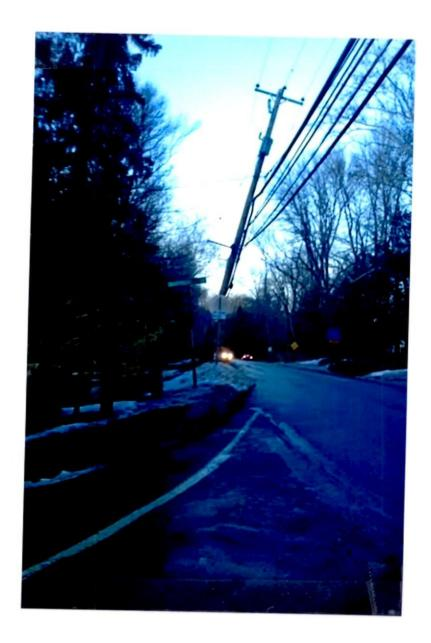
I also have enclosed a photograph of the utility pole at the intersection of Gradyville Road and Bishop Hollow road where the bulk of the trees have fallen on the power lines. Your Honor will clearly see the pole pitched at about a 10-15degree angle and looks like it is about to topple over and is under tremendous stress of having lines running from it at every direction.
