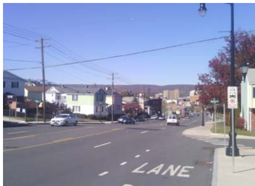
Verizon picture, dead cable and terminal removed
