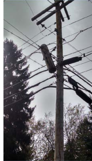
Verizon picture after facilities removed PPL notified to remove pole piece
