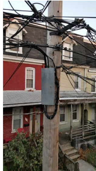
Verizon pictures after VZ work completed, And PPL pole removed, 11/5/15.
