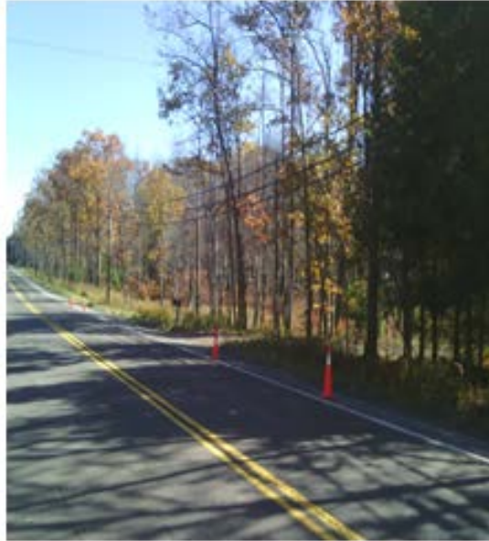
Verizon picture after work completed
