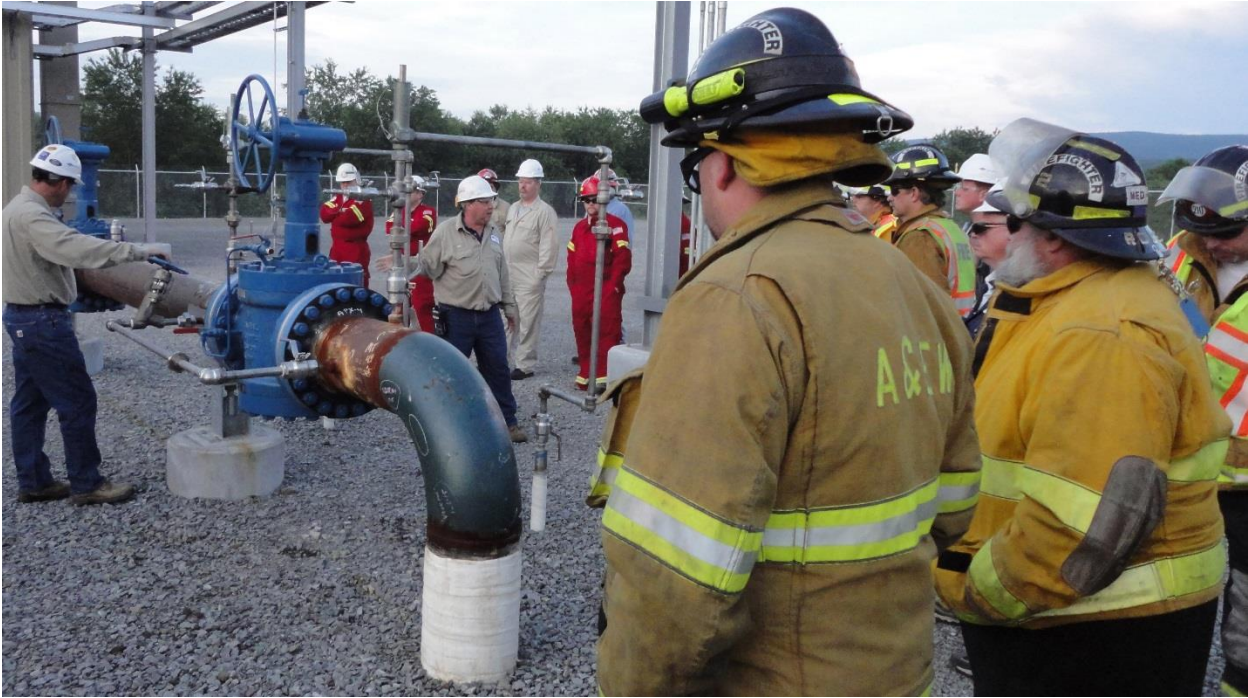
6/18/2015 Cramer Pump Station Orientation & Tour in Indiana County, PA.
