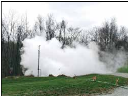
A propane vapor cloud can indicate a pipeline leak.
