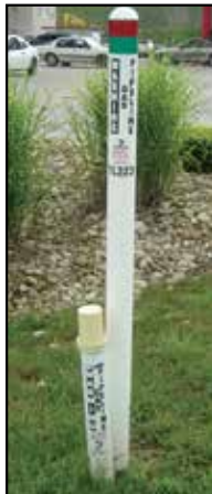
2. linemarker and cathodic protection test station
