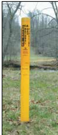
3. high-consequence area entrance or exit marker (arrow on top)
