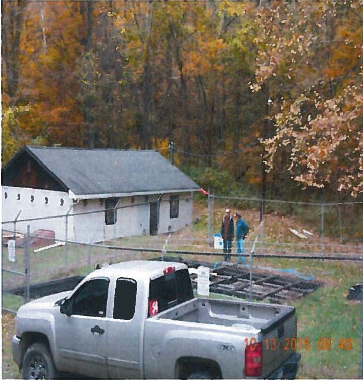
Sewer Treatment Bldg. & Aeration Tanks
