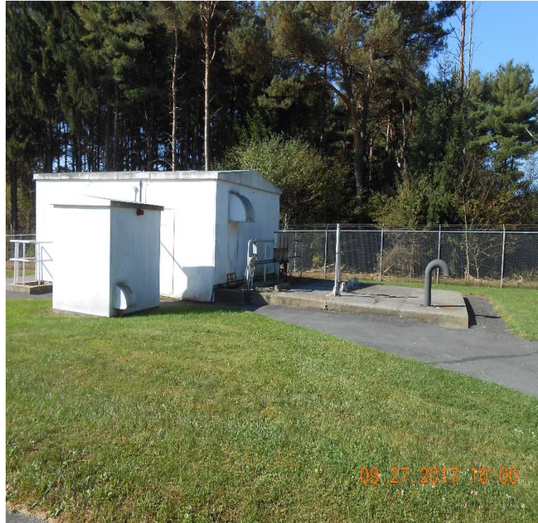
Headwork and Control Building
