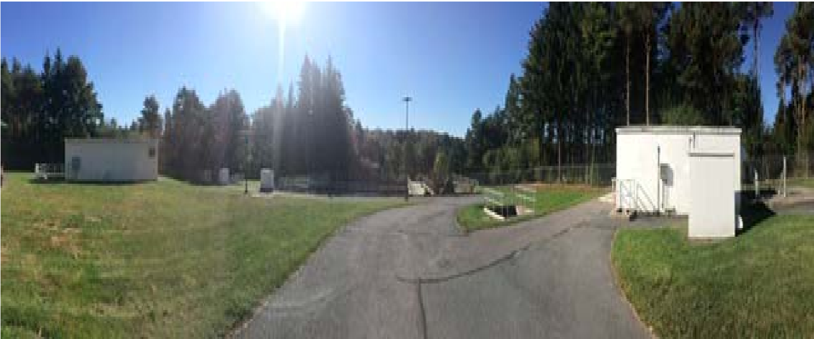
Tobyhanna Sewer Plant
