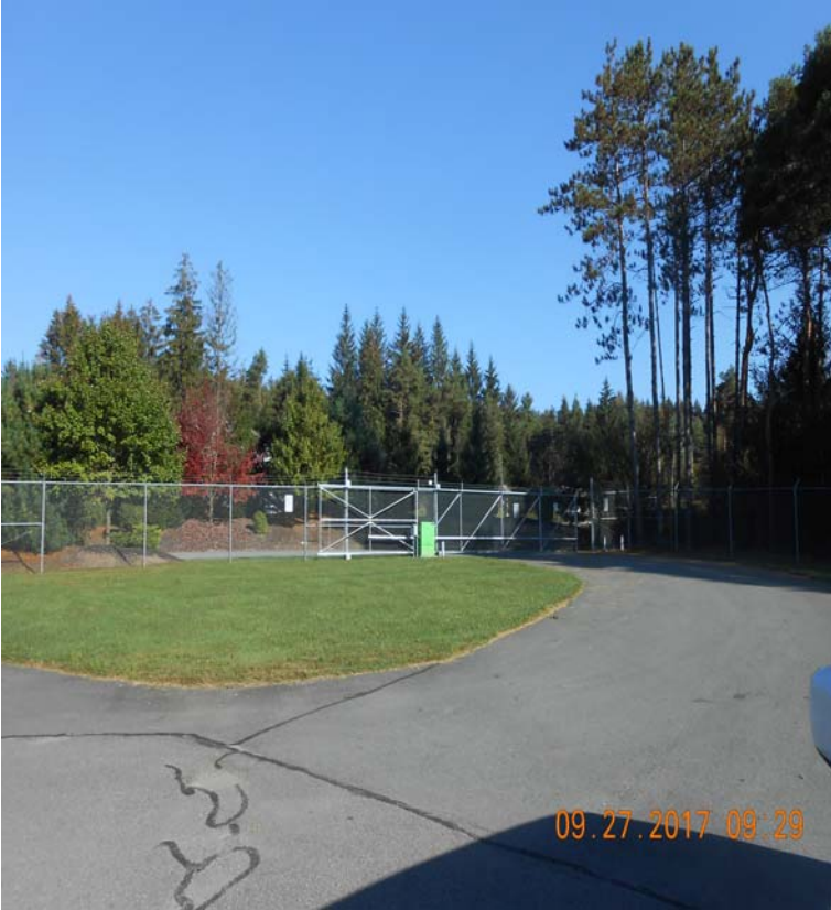
Tobyhanna Sewer Plant Entrance
