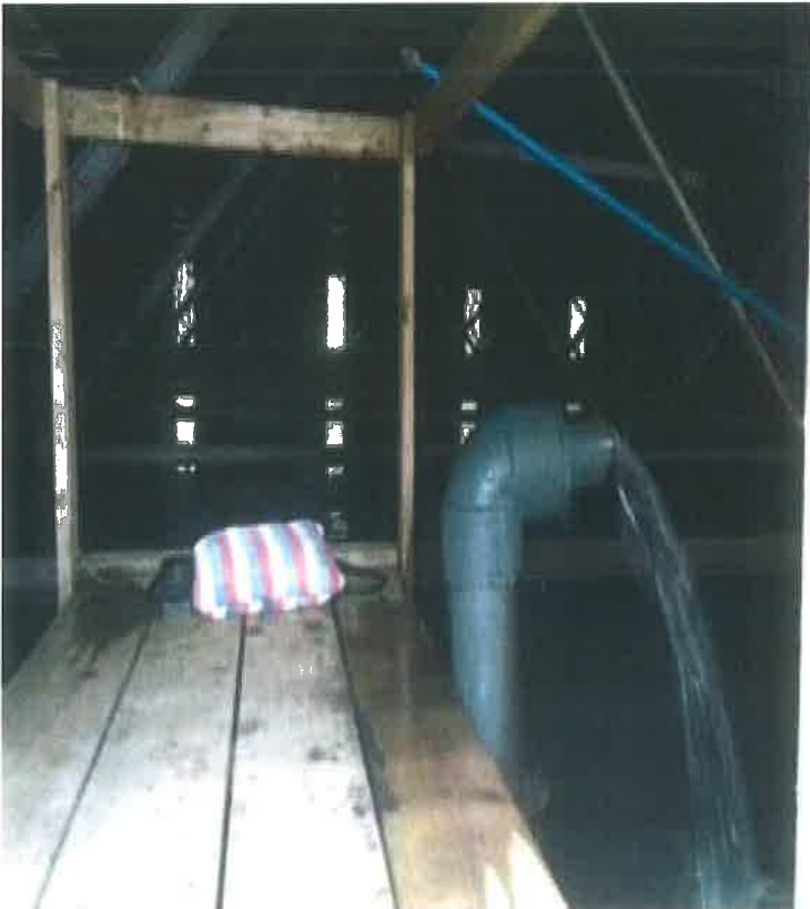
Raw Water Reservoir
