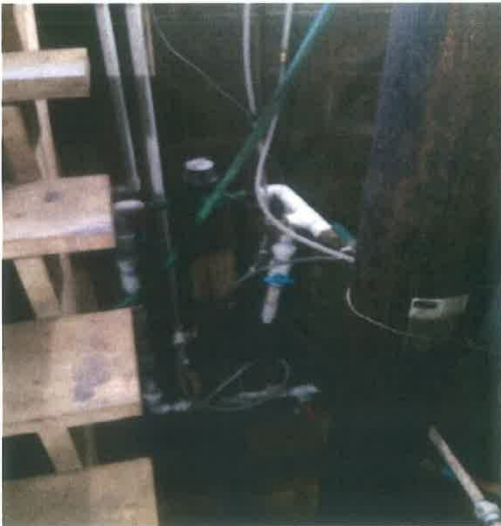
Pipe to Street
