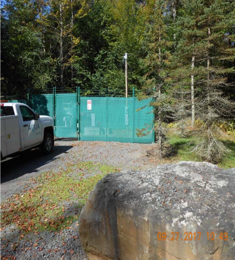
Pump Station #1 – Lady Jennifer
