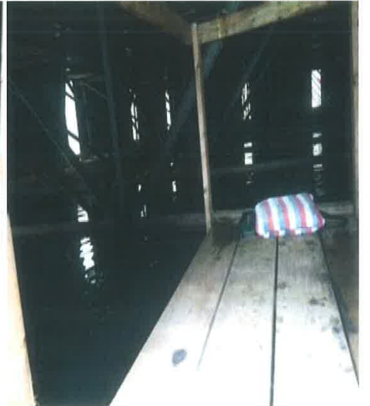
Raw Water Reservoir
