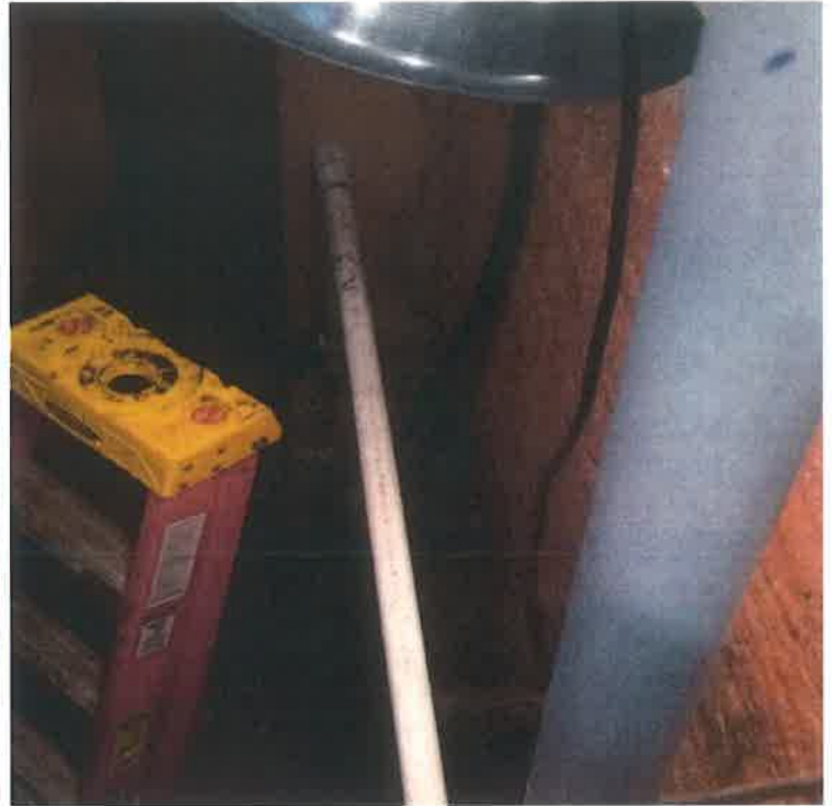
Pipe to Street
