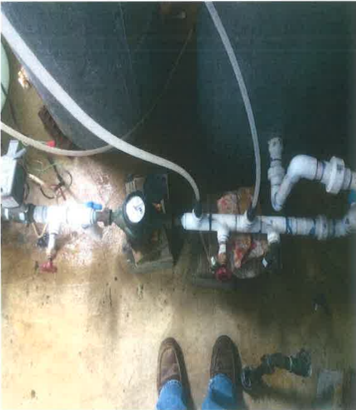
Pipe to Street
