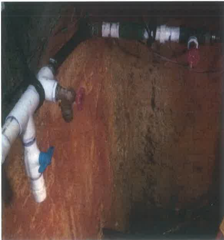
Pipe to Street
