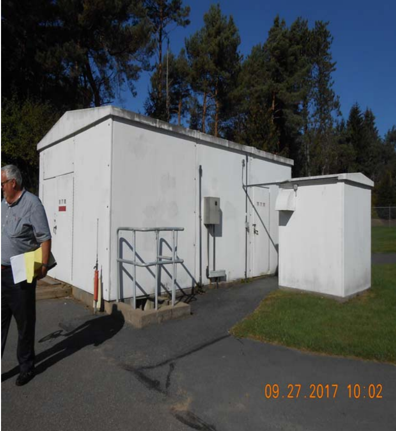
Headwork and Control Building
