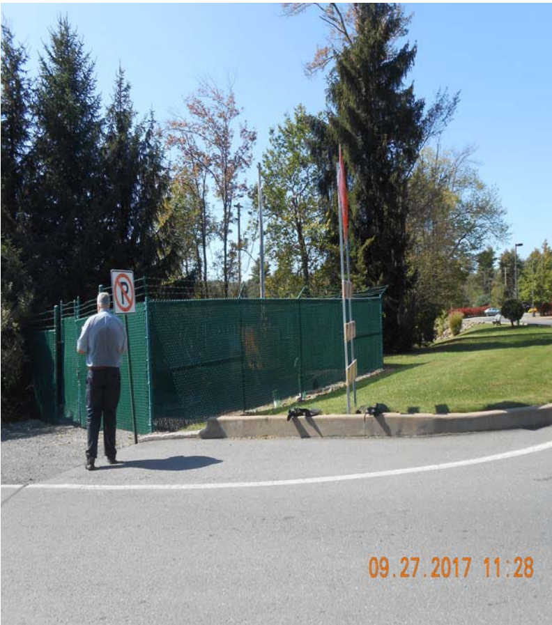
Pump Station #4 – Fernridge
