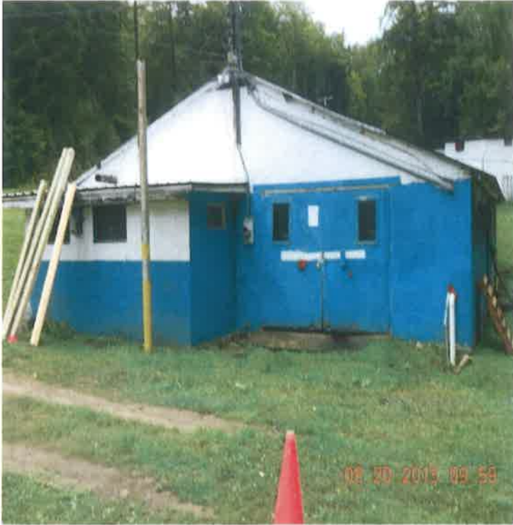
Filter Building (32' x 30' Block)
