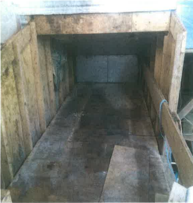
Extra Storage Area
