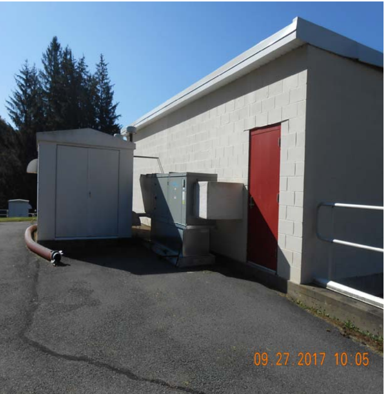
Filter and Blower Buildings
