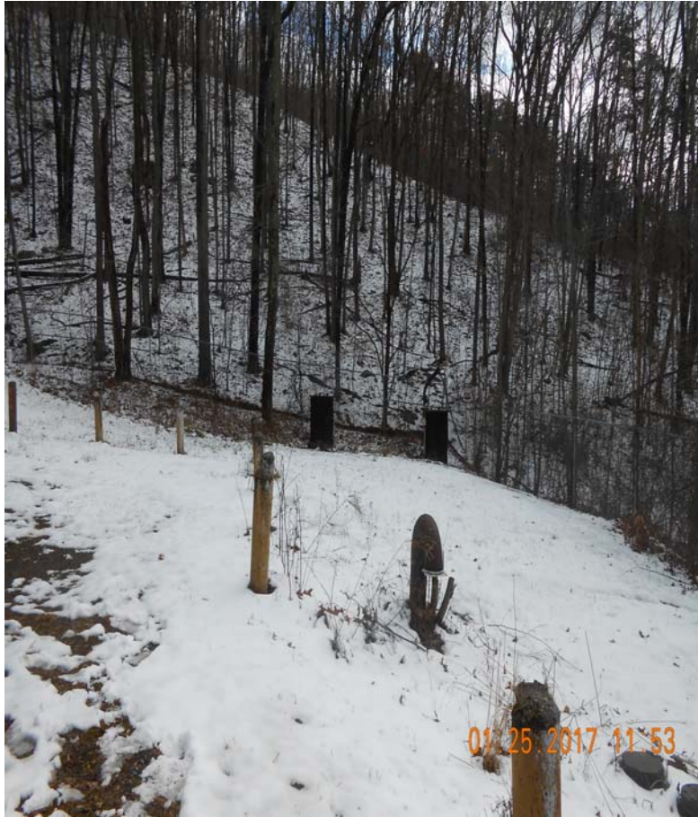
(2) Underground 50,000 gal. Tanks and Well
