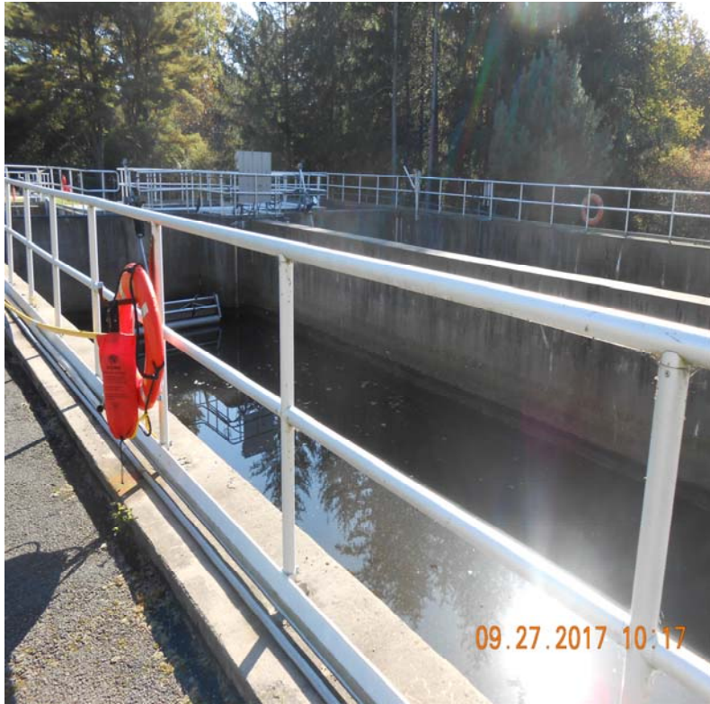
UV Filter Tanks
