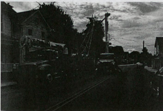
Pulling in New Conductor along Broad Street
