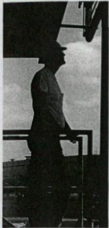
Jerry Howe, Power Supply Supv. Inspects CO Catalyst Change- Out
