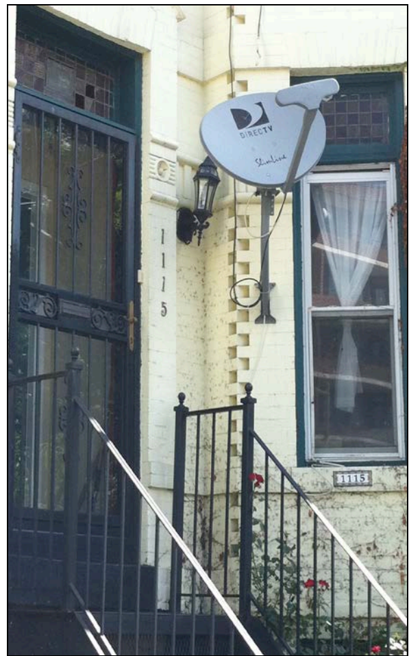
Satellite equipment should not be placed on primary elevations of historic property.
