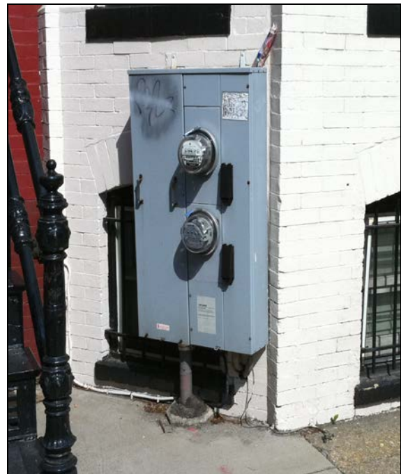
Utility meters should not obscure or cover windows or other distinguishing architectural features.
