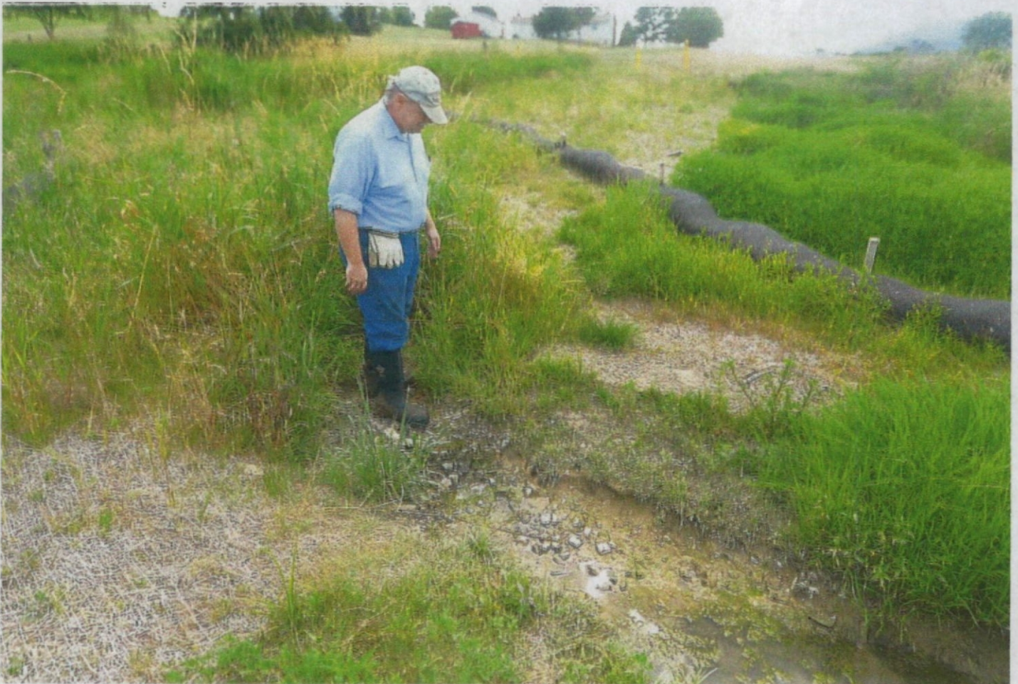
Vern Leach inspects his property where Sunoco Pipeline LP placed a pipeline in Lower Frankford Township.
