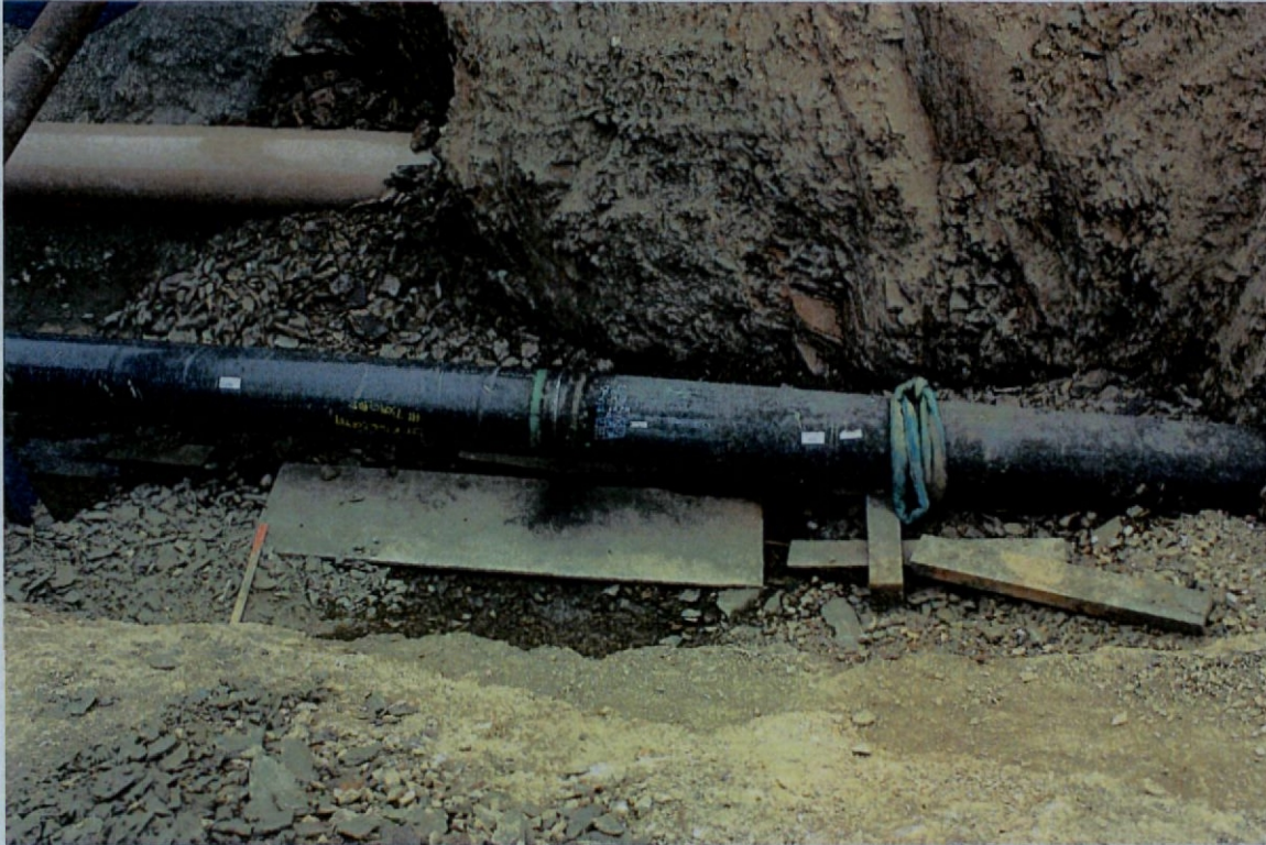
Images taken Sunday May 14, 2017 X70 16" Pipeline in open trench
