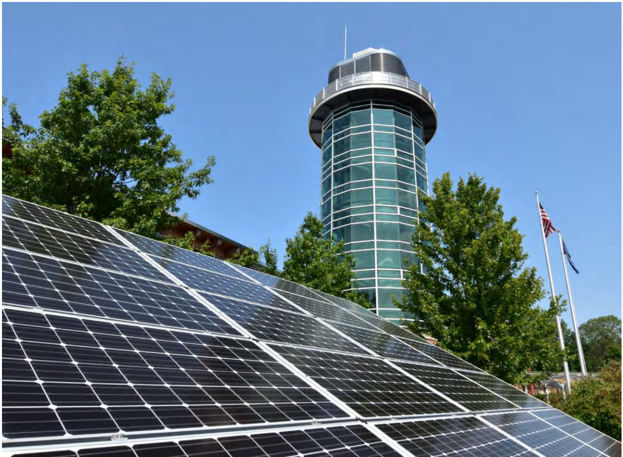
Solar panels at the Tom Ridge Environmental Center, Presque Isle, Erie County
