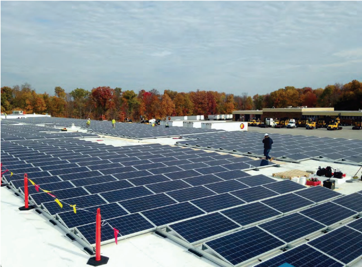
Estes Trucking, West Middlesex, Mercer County
