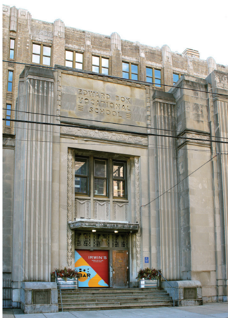
△ Exterior of the Bok Building entrance near 8th and Mifflin Streets.
