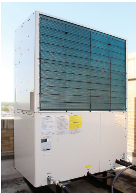
△ 10-ton Yanmar natural gas VRF heat pump located on the Bok Building rooftop.
